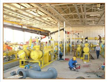
Furthermore, the AFCON SCADA solution monitors the preheating of the water boilers at every PRMS. When depressurized, the natural gas expands and cools down to freezing point which can damage the pressurization valves. Therefore, it is critical to reheat the gas to prevent it from freezing. The AFCON SCADA solution constantly surveys the water temperature at the boilers and reheats water when needed.
